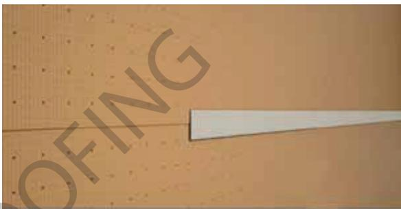
3. Butt join Kingspan AIR-CELL<sup>®</sup> sheets and tape with a 48 mm wide reinforced foil tape.
