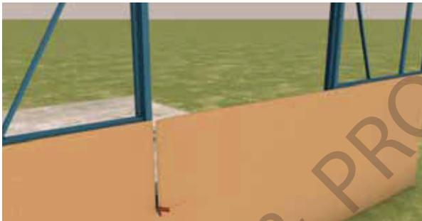
2. Cut Kingspan AIR-CELL<sup>®</sup> carefully around doors, windows and other openings, so that it neatly abuts to frames.
